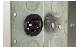
Step 2: Done - Ready for cable.
